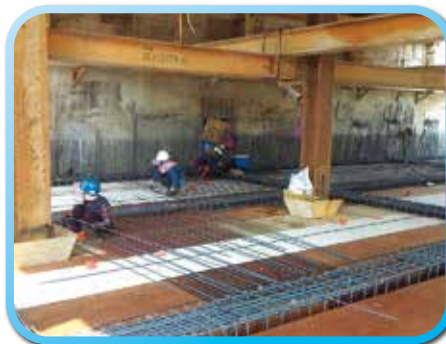
▲ B1FL版鋼筋綁紮
