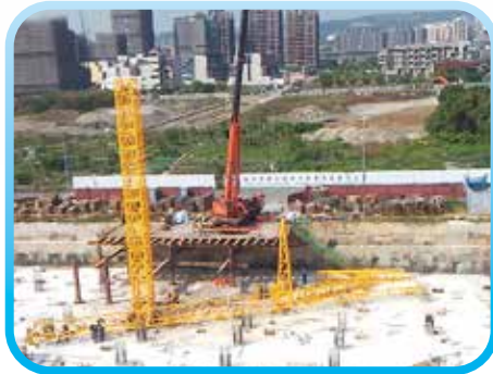
▲ B1FL版鋼筋綁紮
