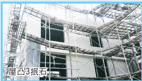
地前後外牆泥作打底已到凸2，室內打底粉光到4樓-2
