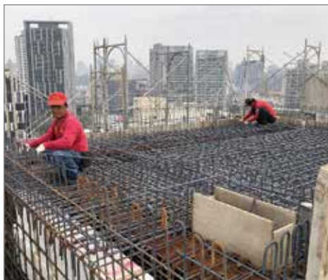
▲屋頂板鋼筋綁紮
